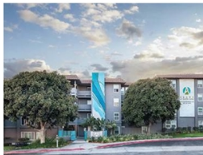
Southern California Multifamily
